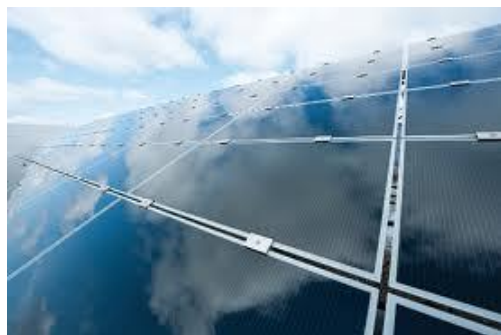
Solar PV Power Plant
