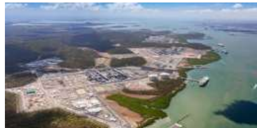
Curtis Island LNG, A legacy of trust
