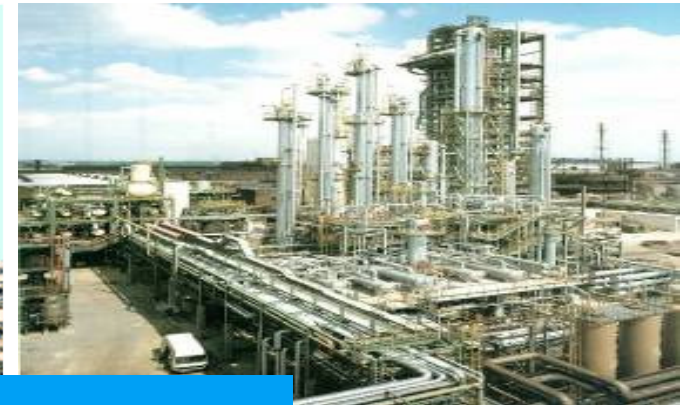
Texaco (GE) coal gasification Oberhausen, Germany coal-to-hydrogen & oxochemicals
