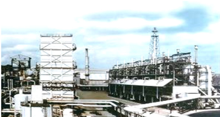
Koppers-Totzek gasification Modderfontein, South Africa coal-to-ammonia/fertilisers
